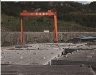
▼ 船盖修理/ Hatch Cover Repair
