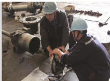
▲ 艏側推修理/Bow Thruster Overhauling
